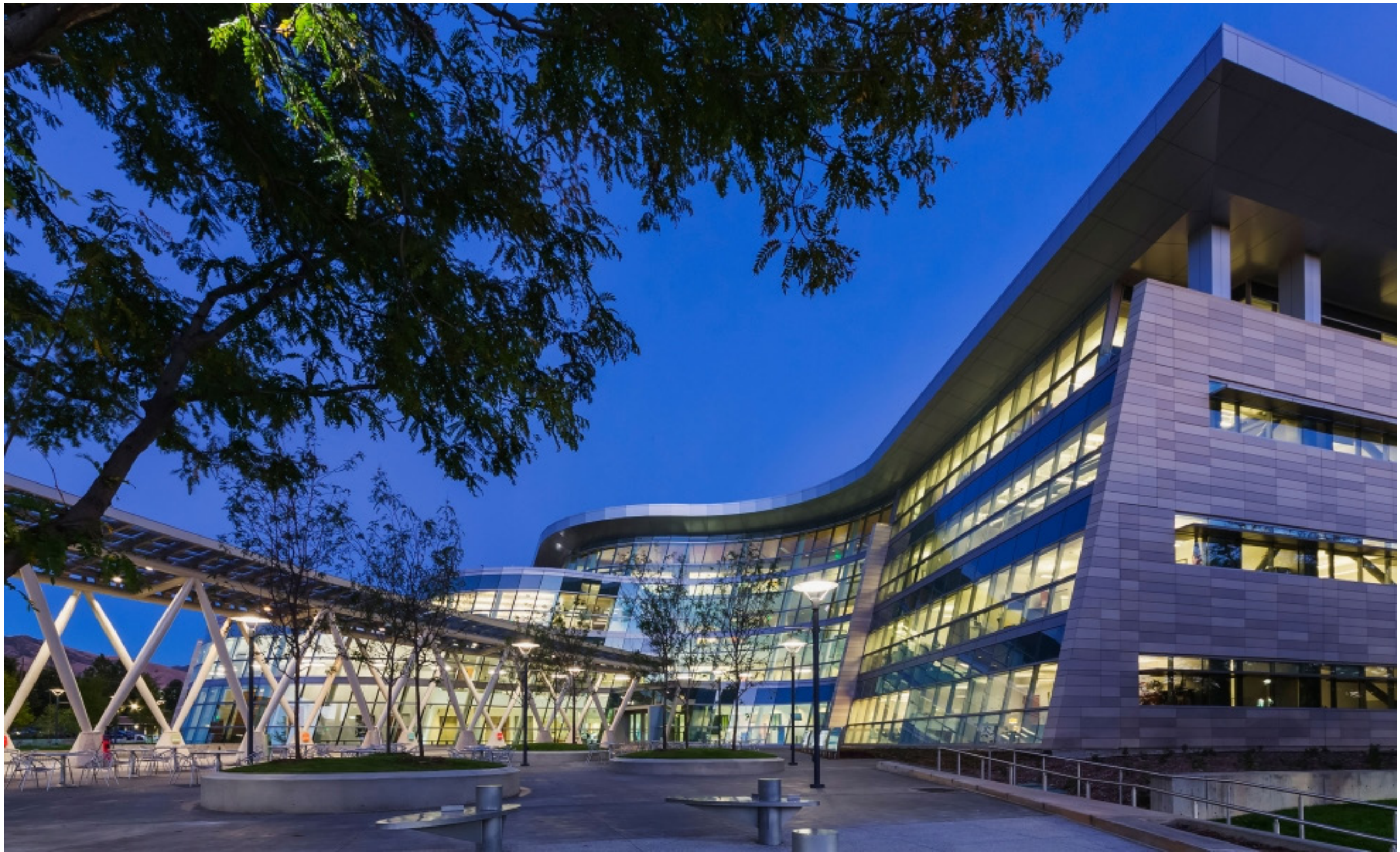
SALT LAKE CITY PUBLIC SAFETY BUILDING
